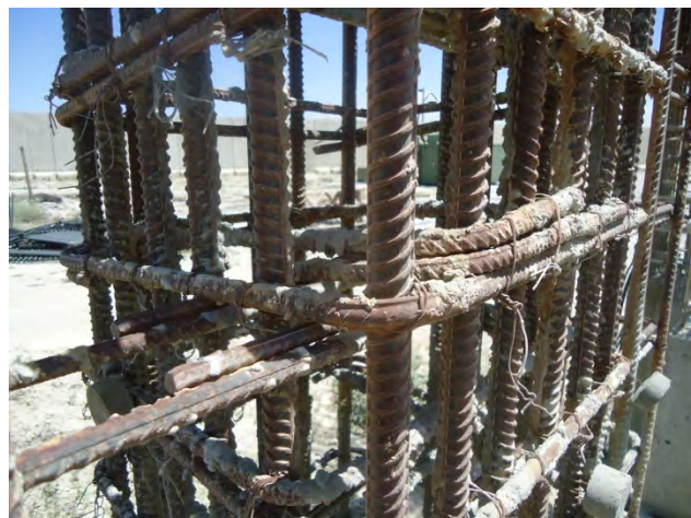
Photo 3 - Rebar Is Tied Together Instead of Welded
