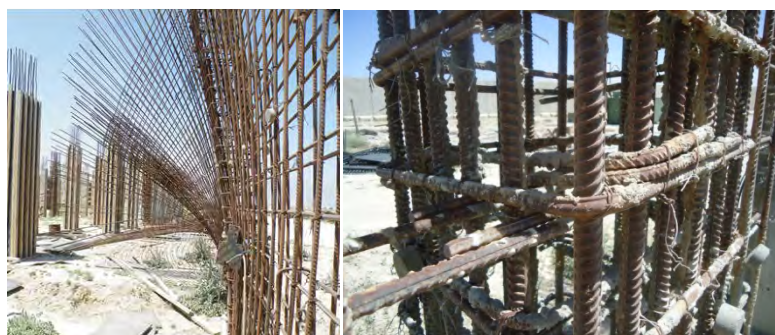
Tilted columns, sagging reinforcing rods, and faulty rebar at the JCIP courthouse construction site in Parwan province, Afghanistan.
