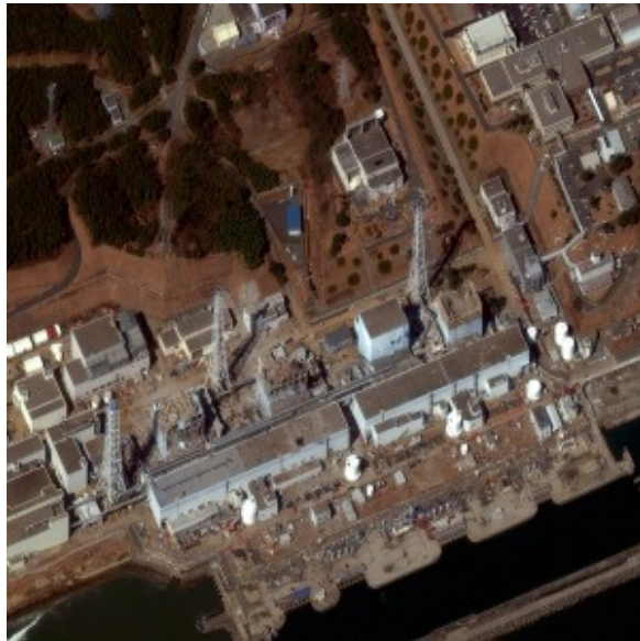
Damage at Fukushima Daiichi as seen on March 18, 2011. (photo: DigitalGlobe)
